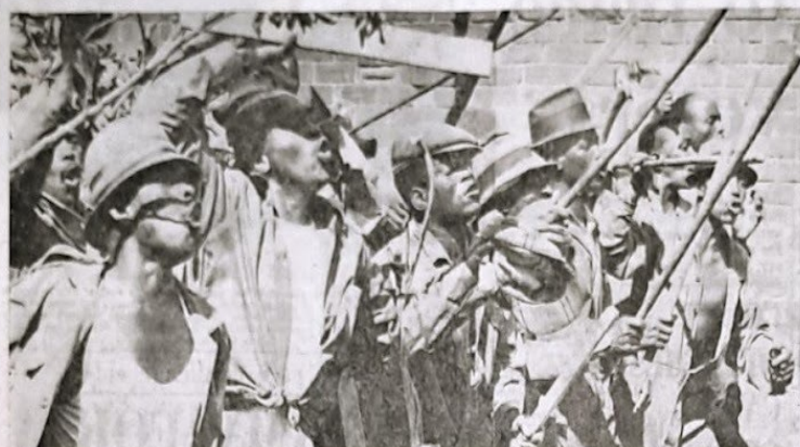
BRANDISHING sticks — and anything else they could lay their hands on — a chanting mob of African workers of the City Engineer's Department marches down Old Fort Road in impetuous today to gather outside the department's headquarters to demand higher wages.
